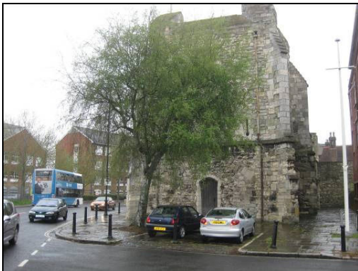
Photo 2.3: tree T4 (north side of road)
