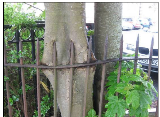
Photo 2.8: Structural weakness in T12
